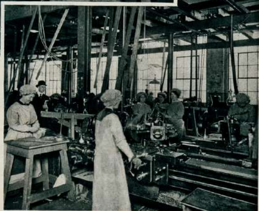
Rough turning the Adaptor Second operation
