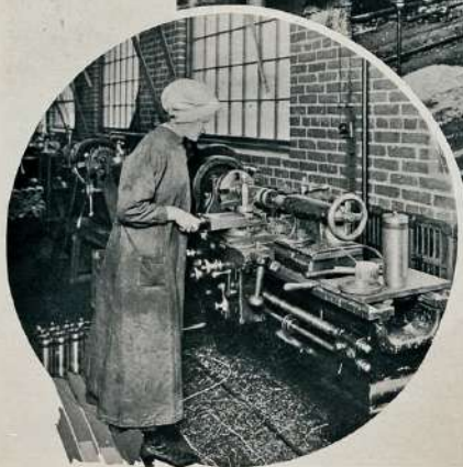
Finish Turning and Profile 18-pounder Shrapnel.
