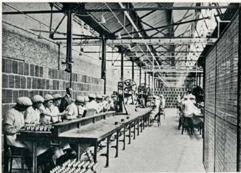
Finished Assembly No. 80 Fuse
