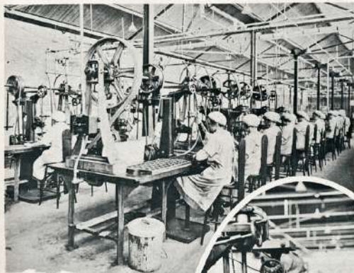
Finishing the Top Ring of No. 80 Fuse
