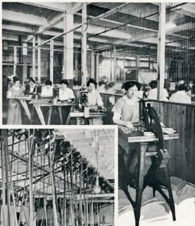
Foot Presses. Pressing Needles in Needle Plug.
