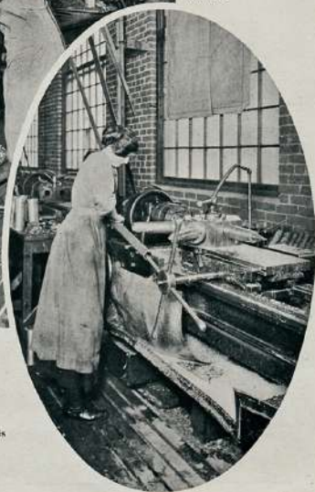
Chambering or Boring 18-pounder Shrapnel
