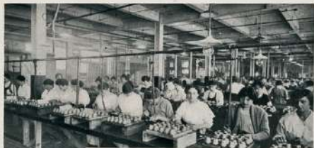
Assembling No 100 Fuses
