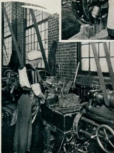
Turning Copper Driving Band, 18-pounder Shrapnel
