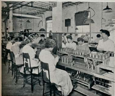
Inspection of Top and Bottom Rings No. 80 Fuse
